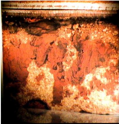
Example 3 Inside Mild Steel Pipe
